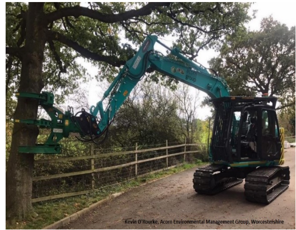
Fig 14: A tree shear mounted on an excavator or tractor can delicately extract trees from dense broadleaved woodlands
